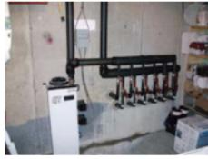
The old, inefficient heating system was this hybrid (above left) that burned both wood and fuel oil. It was replaced with this water-to-air ground-source heat pump (right) which passes water over a heat exchanger to heat the air that warms the house. The picture above shows the QT pump control that controls the loops consisting of six supply lines and six return lines — pipes that run underground below the frost line to absorb or dissipate heat.
