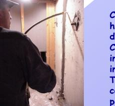
Concrete cracks, construction joints, tie-rods, honeycomb sections and all other types of joints of deficiencies can be permanently sealed using our Chemical Grout Injection process. This professionally installed system is designed to completely stop the leak in the concrete by creating a flexible, gasket-like seal. The resin is pressure pumped (picture at left) into the concrete using specialized equipment to ensure complete penetration of the grout.
