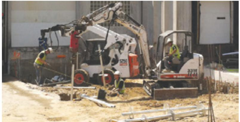
Skid-steer and mini-excavator installing helical piles
