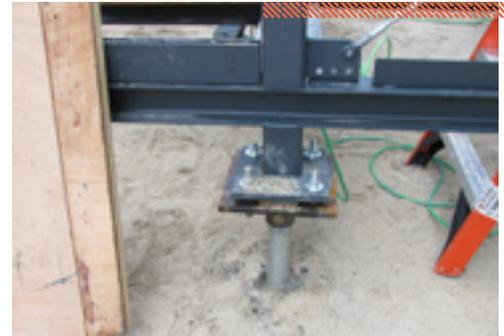
Beach house framing bolted to helical pile
