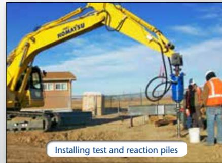
Installing test and reaction piles
