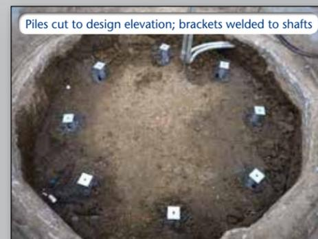
Piles cut to design elevation; brackets welded to shafts
