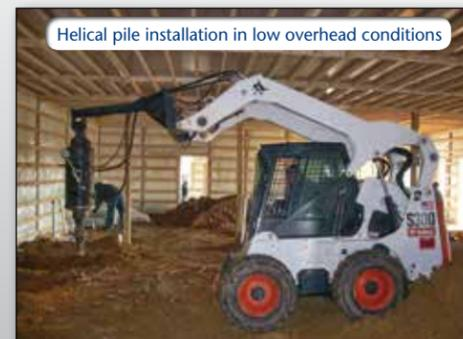
Helical pile installation in low overhead conditions
