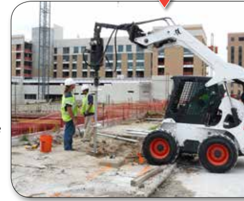
Helical piles to support crane pads at a construction site
