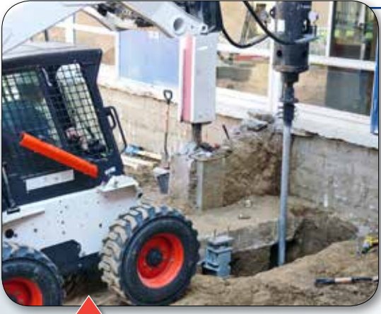
Retrofit helical piles to support an existing column at a school
