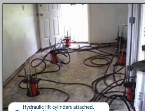
Hydraulic lift cylinders attached. The slab and interior non-load bearing walls are lifted back to a level position.
