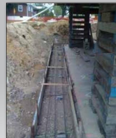
Rebar is placed over installed new construction piers. The footing is ready for concrete.
