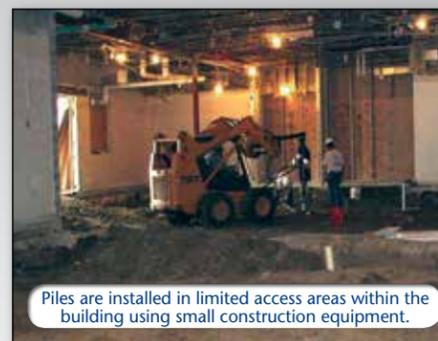
Piles are installed in limited access areas within the building using small construction equipment.
