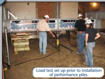
Load test set up prior to installation of performance piles.
