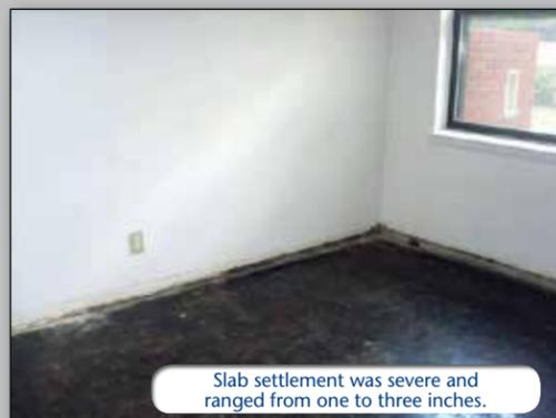
Slab settlement was severe and ranged from one to three inches.
