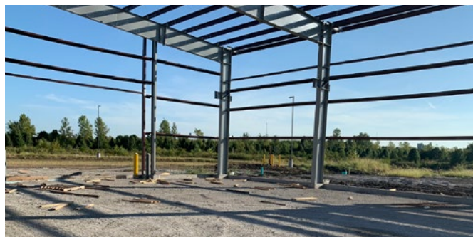
Building shell erected
