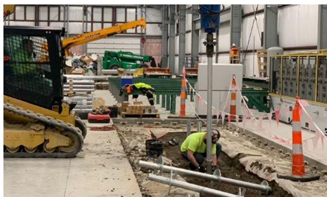
Phase 1 helical piles being installed
