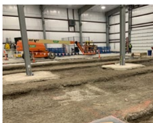
Phase 2 area prepared for pile installation around spread footings
