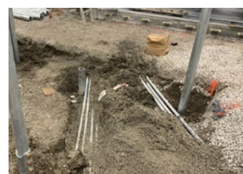
Installing helical piles around existing utilities (Phase 2)
