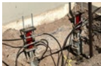
Lift cylinders attached to brackets
