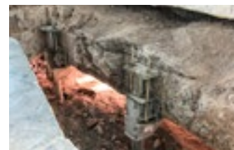
Lifted structure with brackets locked in final position at Southeast corner
