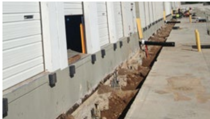
Piers installed along the east wall
