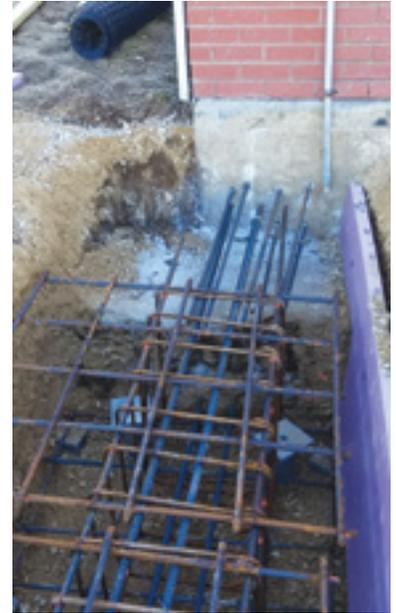
Pile cap and grade beam reinforcement installed around helical piles
