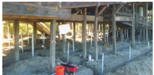
Helical piles installed within grade beams at column locations
