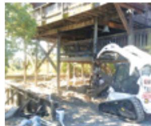
Predrilling at column locations prior to helical pile installation
