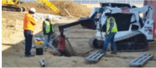
Installing helical piles with a skid steer
