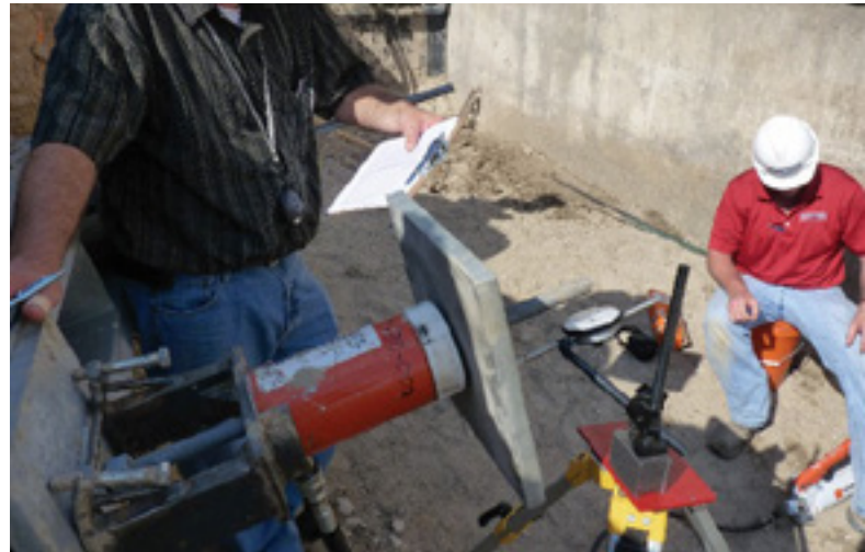
Proof test on a tieback anchor
