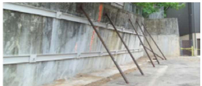
Completed tieback and waler system prior to removal of temporary bracing
