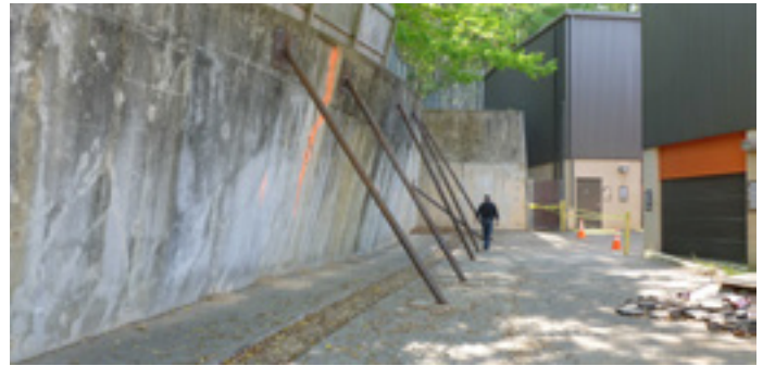
Retaining wall temporarily stabilized with steel tube bracing
