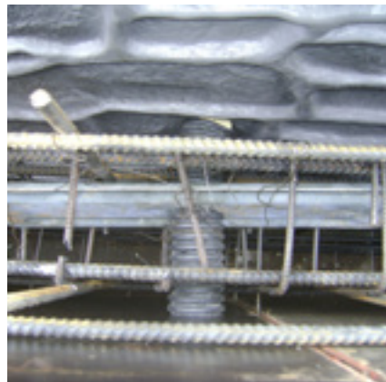
Top view of bearing plate inside the reinforcement
