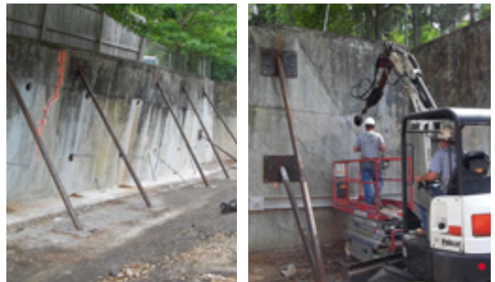
Bottom row of helical tiebacks being installed around bracing
