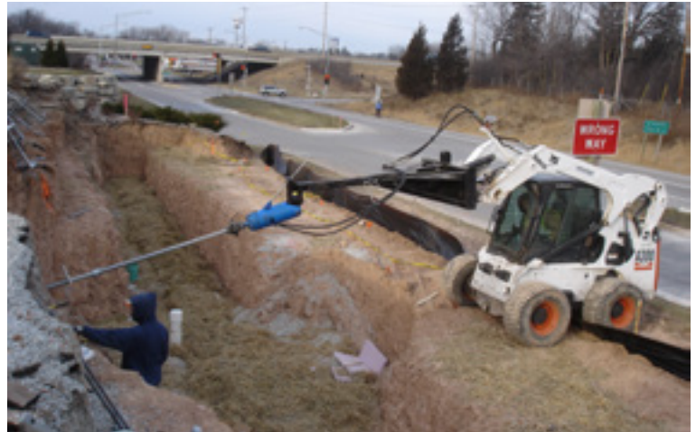
Helical tiebacks installed with a skid steer
