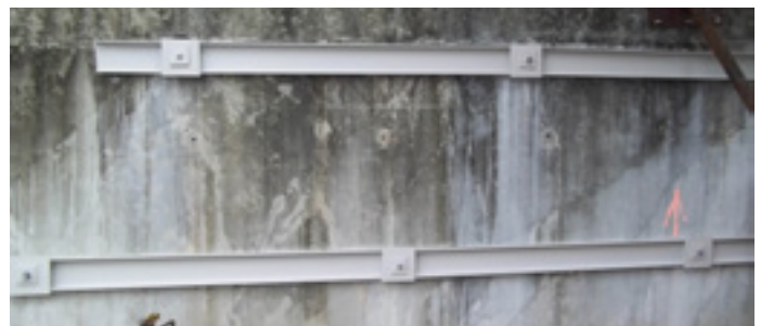
Top and bottom tieback and waler system in place
