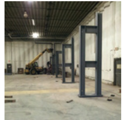
Columns supported by helical piles
