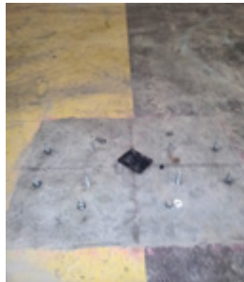
Pile caps poured flush with slab for crane columns
