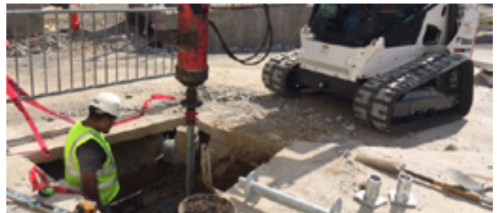
Skid steer used for installation
