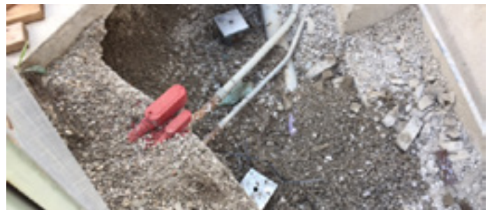
New construction brackets in place
