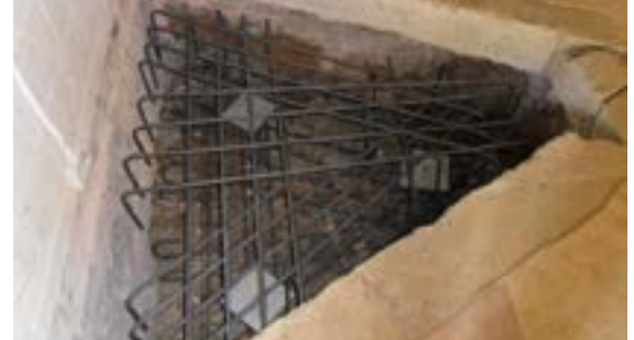
Installed piles capped and rebar placed to pour footing
