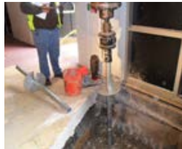
Advancing helical pile
