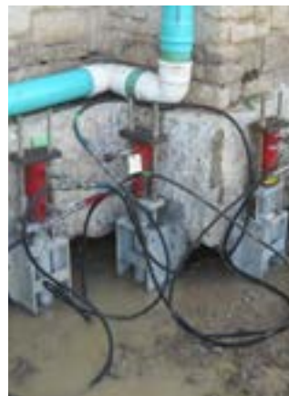
Lift cylinders fitted to installed piers
