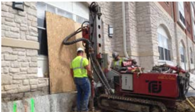
Pre-drilling at production pier location
