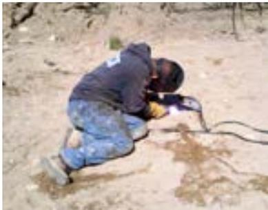
Piles cut to design elevation and new construction brackets tack-welded in place
