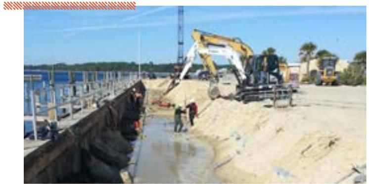
Excavation made behind seawall for tieback installation
