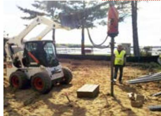
Advancing lead section of 3.5-inch O.D. pile
