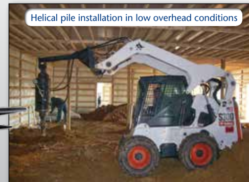
Retrofit pile systems used to re-level structure
