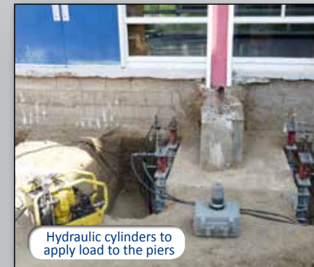
Advancing helical piers adjacent to existing column footings
