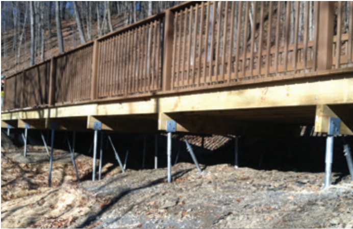
Boardwalk supported on 2.375" O.D. vertical and battered helical piles
