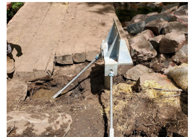
Piles, anchors, and brackets installed
