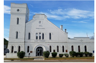
Fort Coombs Armory
