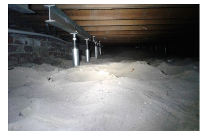
SmartJacks installed and attached to new support beam
