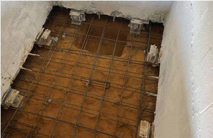
Reinforcement installed in new floor location
