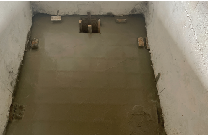
New concrete floor poured
