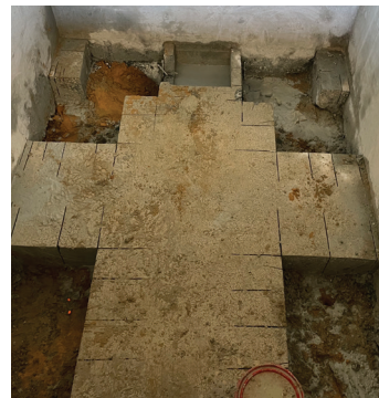
Elevator shaft with floor removed at underpinning locations
