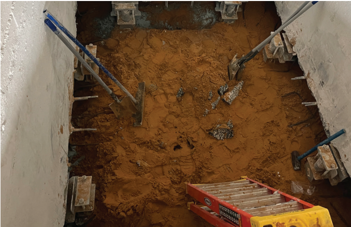
Retrofit piers and brackets installed with floor removed
