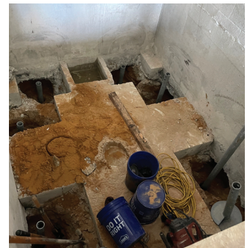
Installing helical piers from above
