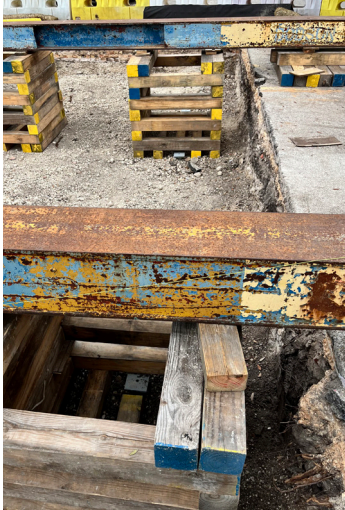
Cribbing and beam tracks placed above helical piers
