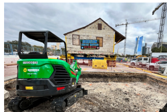
Excavating relocation area for helical piers
