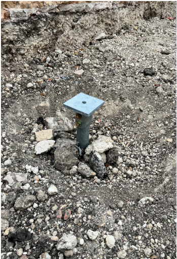
Helical pier with new construction cap installed
