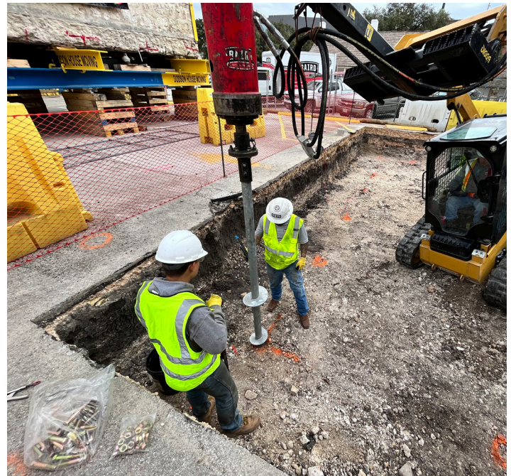
Installing helical piers
