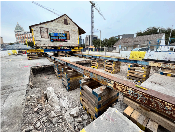
System for moving structure to support locations
