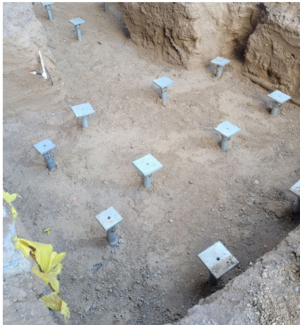
Additional helical piles installed to increase capacity
