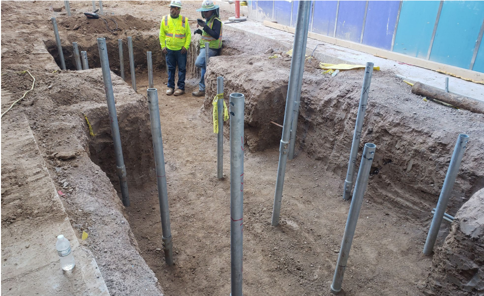
Helical piles installed in pile cap excavation
