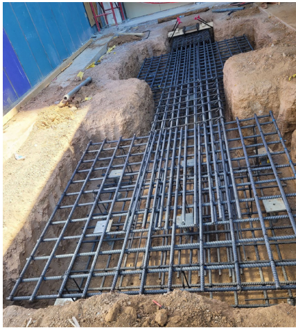
Reinforcement installed around helical piles
