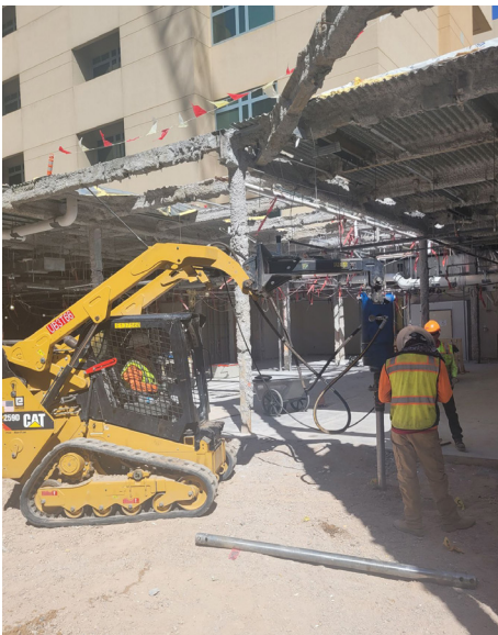
Installing helical piles
