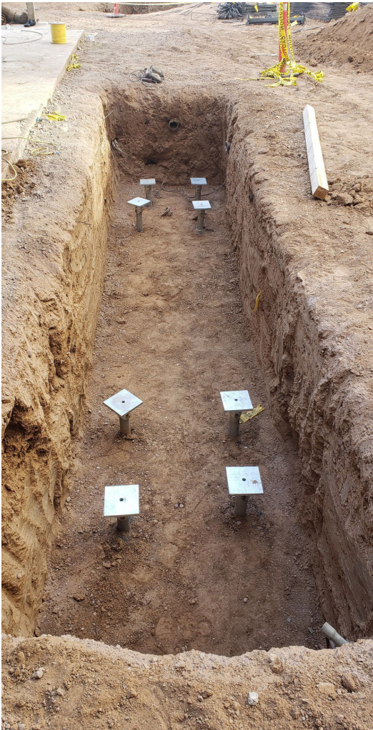
Helical piles with new construction brackets installed
