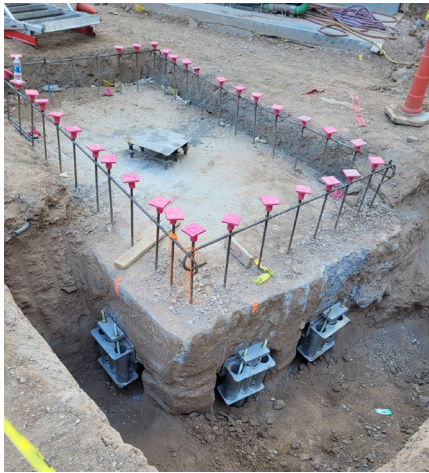
Concrete pile cap with retrofit helical piers installed
