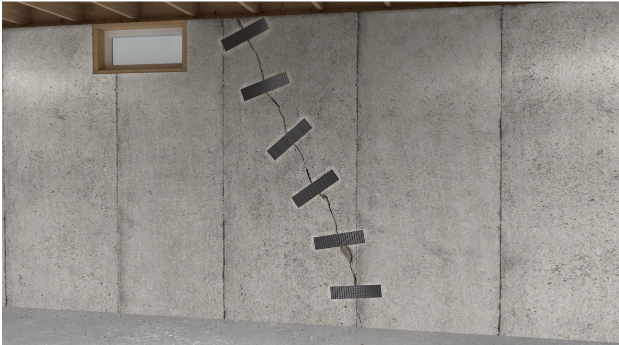
Rendering of the CarbonArmor® Wall Stitch system installed within a basement
