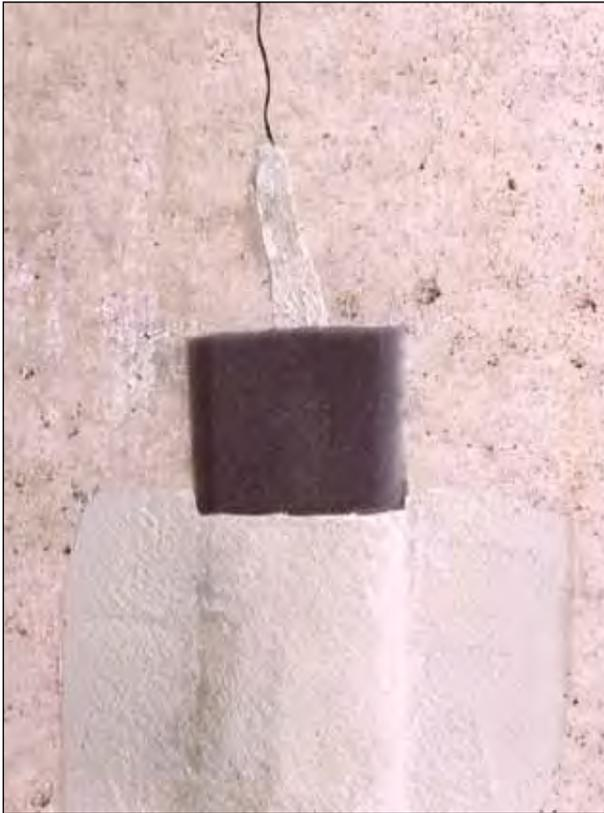
It's important to remember that the FlexiSpan® System is not draining much water at all since it incorporates a seal first! If it ever allows any water through the first seal, it would only be less than 5% of the original seepage. The drainage component is an innovative second line of defense to handle this minor seepage, if it ever occurs. This is what makes FlexiSpan® a special repair with completely predictable results:
